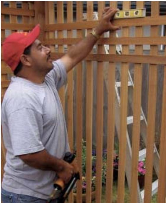
**Figure 4. Site-built privacy screens add a custom touch. They're made with the same material as the deck, and assembled with stainless steel staples.**
