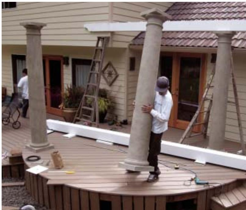
**Figure 8.** Fiberglass arbor and pergola kits are available to create a classical or Tuscan look. These hollow columns anchor to the deck framing using a length of all-thread.
