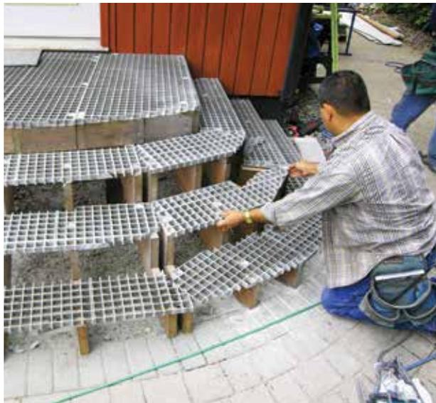
**Figure 2.** The fiberglass grating panels can be cut to fit with a circular saw. Here, the deck surface fits just beneath the door threshold, with the framing sloped slightly away from the house for drainage.
