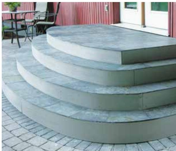
**Figure 8.** The tiles were butted closely together and installed without grout, allowing water to drain between the tiles and through the fiberglass grating.
