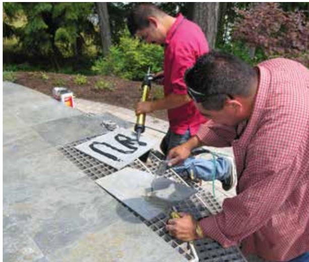
**Figure 5.** To ensure good adhesion, each slate tile was washed off with water, thoroughly dried with compressed air, and wiped down with denatured alcohol before glue application and installation.
