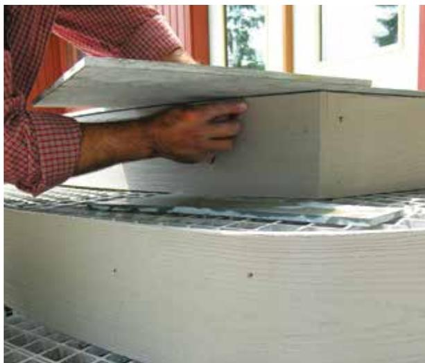
**Figure 7.** At the edges of the deck and the steps, the tiles needed to be scribed, then cut to fit with a wet saw.
