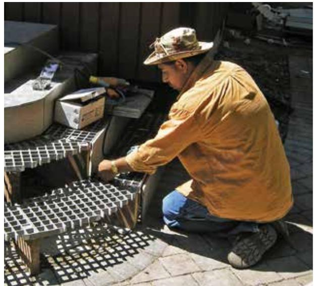
**Figure 3.** Cellular PVC trim was used to form the curved fascia trimming the stair risers. A heat gun was needed to warm up the trim and make it flexible enough to bend around the tight curves. When heating and bending PVC lumber, keep the gun moving to avoid blistering the trim.
