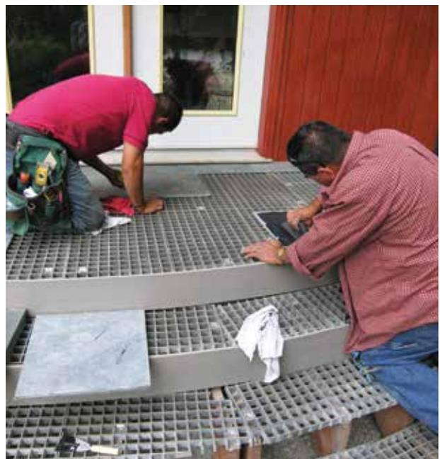
**Figure 4.** The author planned the framing and the tile layout so there would be full tiles, rather than small cut pieces, along any edge. Anywhere that tiles needed to be cut, no piece was narrower than 4 inches.
