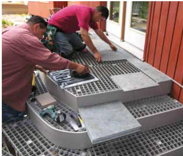
**Figure 6.** The tiles were glued to the fiberglass grating with a structural adhesive, which was applied to the back of the tile with a caulk gun and then spread with a V-notch trowel.
